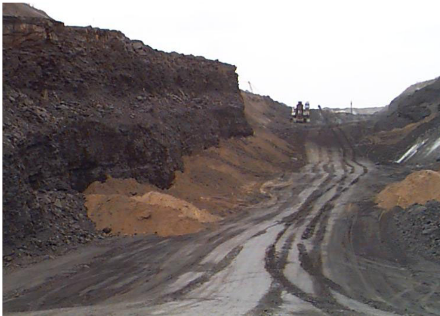
Figure 17: Open bords sealed by sand cladding
