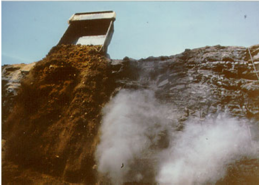
Figure 16: Cladding by tipping over the highwall
